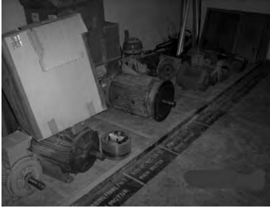
Proper house-keeping of the electric motors.
