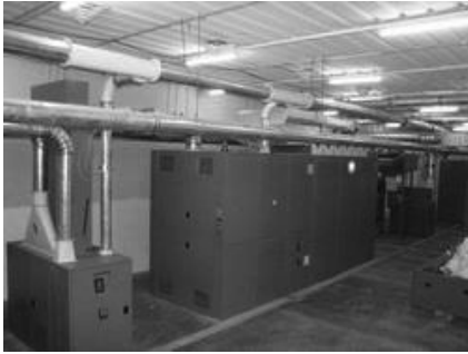
Centralized waste unit collect wastes from different machines in blow room
